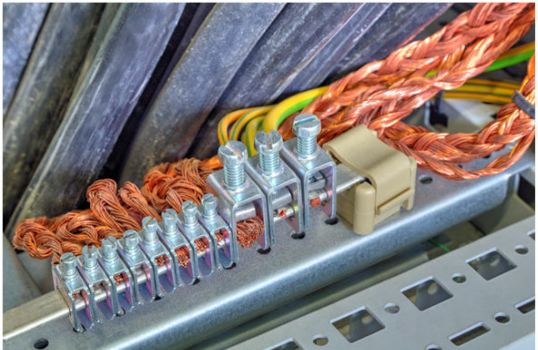
Grounding terminals and wires. (Image by phadventure © 123RF.com.)
